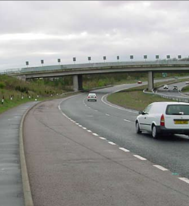
An unprotected lay-by on a right-hand bend is often mistaken for the main carriageway
