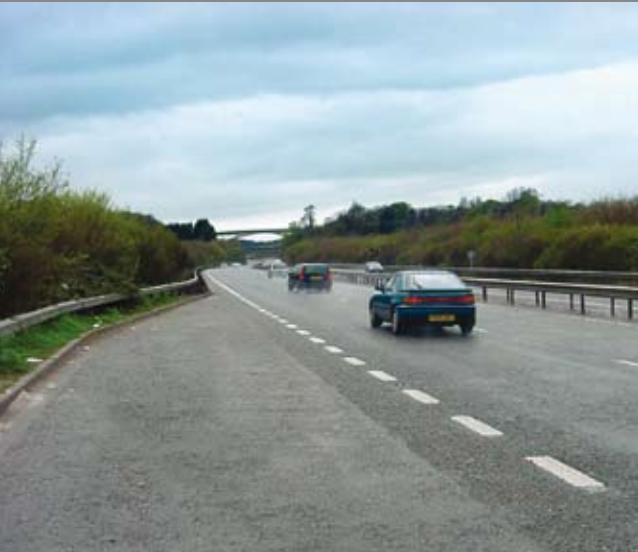
An unprotected lay-by on a two-lane dual carriageway
