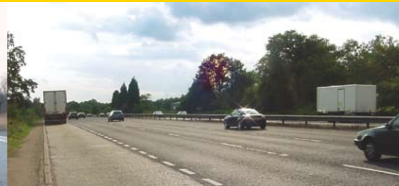
An unprotected lay-by on a three-lane dual carriageway
