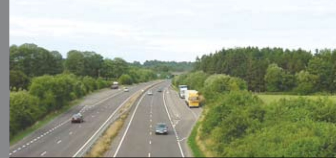
A kerbed island gives lay-bys greater protection
